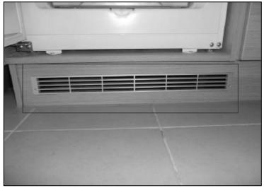
IMPORTANT: The appliance aperture MUST have a minimum of 200 cm<sup>2</sup> free air flow for ventilation.
