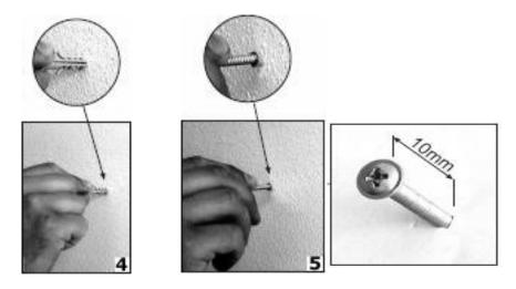
4) Insert raw plugs into all of the holes that you have drilled.
