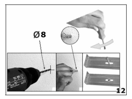
**12)** Using a 8 mm drill bit, drill out two holes on the pencil markings that you made in step 11. Insert raw plugs into the holes and then use a screwdriver to secure the fixing bracket to the wall.
