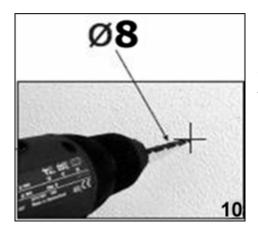
**10)** Remove the hood from the mounting bar and then using a drill bit with an 8 mm diameter, make holes in the wall on the positions that you marked in step 9.
