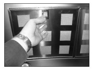
**1)** Remove the metal grease filters.
