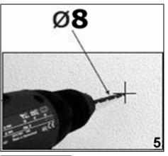
**5)** Using a drill bit with an 8 mm diameter, make holes in the wall on the positions that you marked in step 4.
