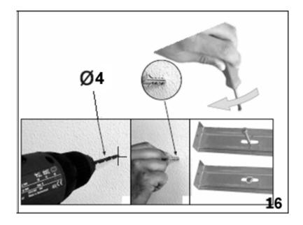
**16)** Using a 4 mm drill bit, drill out holes on the pencil markings that you made in step 15. Insert rawl plugs into the holes and then use a screwdriver to secure the fixing bracket to the wall.
