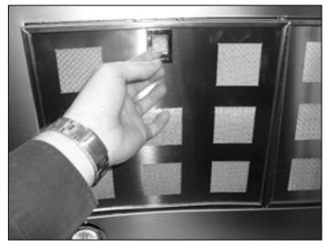
Remove a grease filter by lifting up the catch and then pulling the filter away from the hood.
