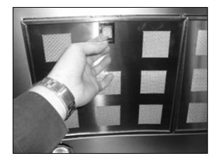
Remove the grease filters.
