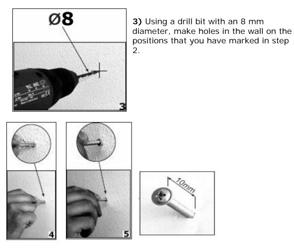
4) Insert rawl plugs into all of the holes that you have drilled.
