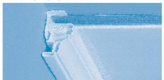
Fit wall boards flush with ceiling. \*Spot drill through mounting strip and wall board at regular intervals. Drill out the wall and fit wall plugs flush with the surface of the wall board. Fix the mounting strip using flat head screws. Fit the ceiling boards and finish by clipping the front face of the cornice into place.
